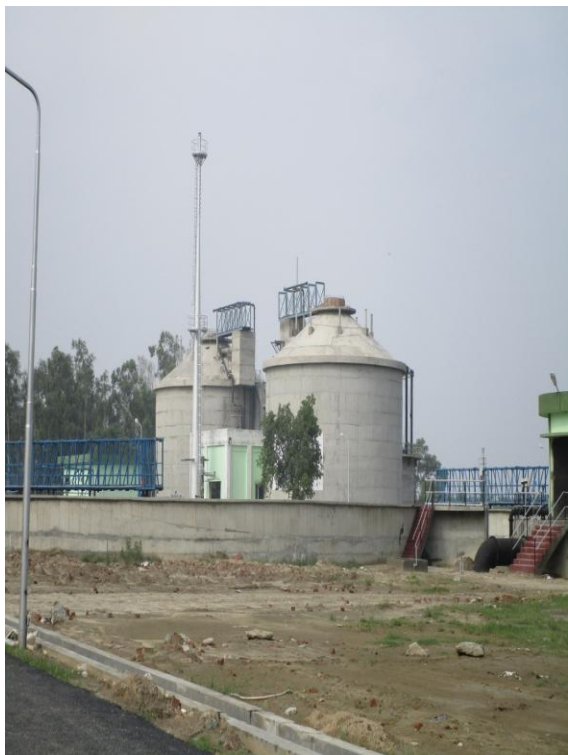
ANAROBIC SLUDGE DIGESTER:-
